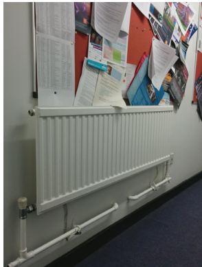
(c) The central heater which emits strong magnetic reading up to 80 \mu\text{T}
